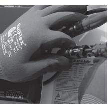
PRE-INSTALL MLPE: Install MLPE in a location on the module that will not interfere with microrails or grounding lugs. To use trunk cable most efficiently, install MLPE components in the same locations on all modules in the same row.
